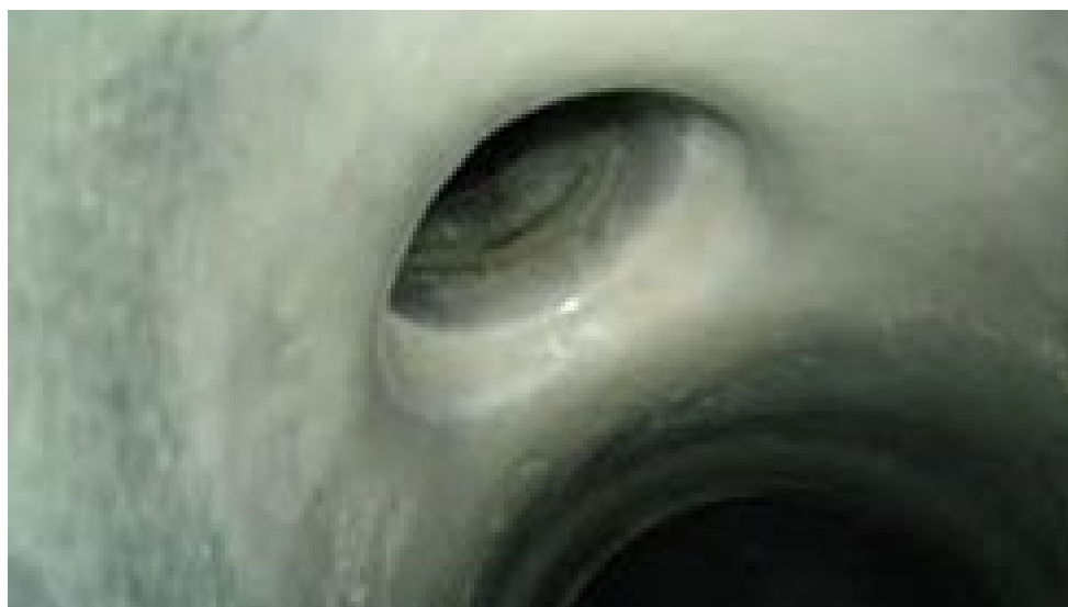
Top hats installed at laterals
